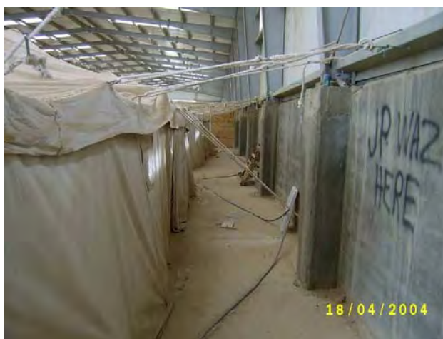
Figure 2. Generator Cable and Housing Unit Involved in Specialist Campo-Siles Electrocution (From Army Photographs)
